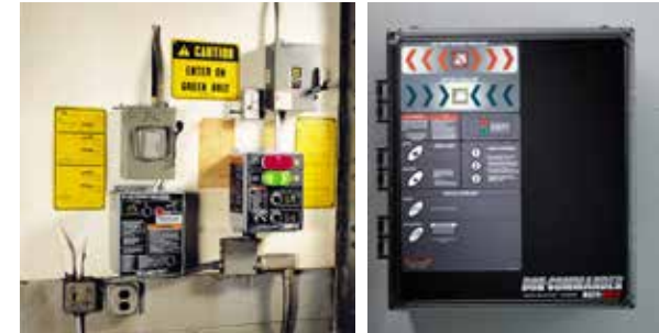
Multiple controls at each dock position can be complicated and potentially dangerous.
