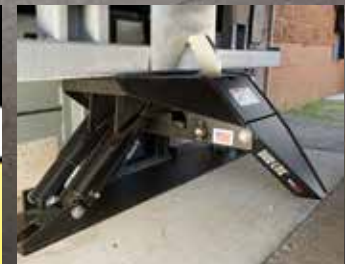
Stabilizing Trailer Restraint with cover plate obstruction
